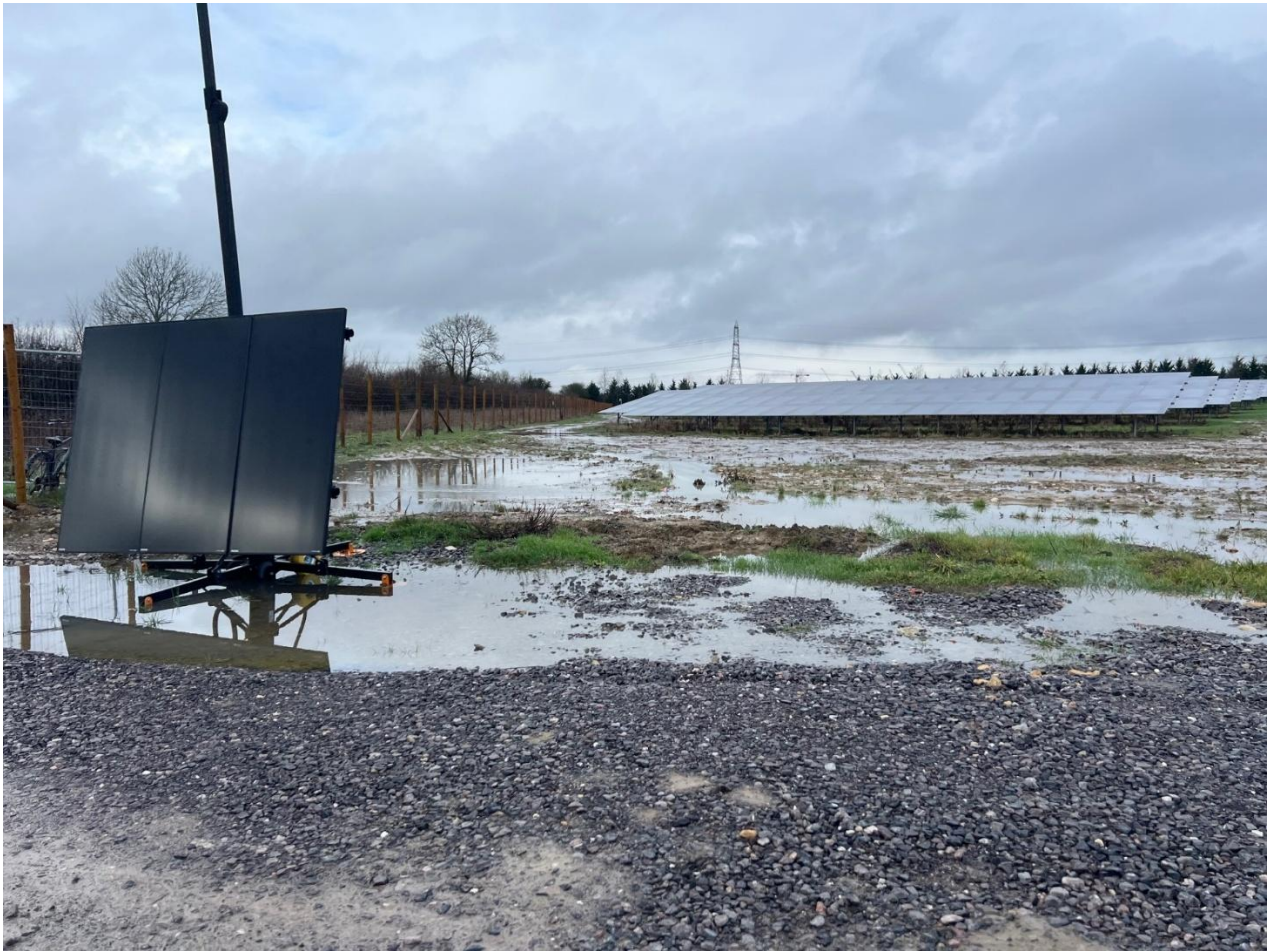
Flooding due to construction compaction and subsequent run off
