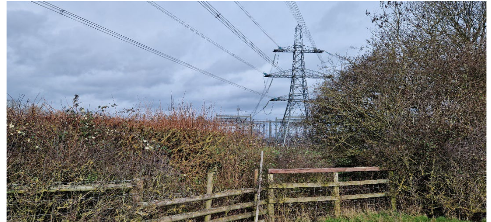
View from proposed diverted route of ECL4/2 behind E/Claydon substation.
