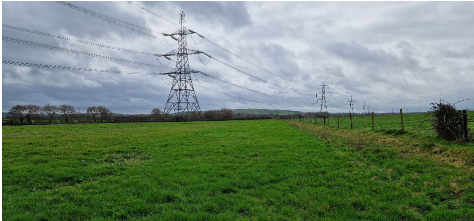
View from junction of ECL/3/2 and ECL/4/2 towards Botolph Claydon.
